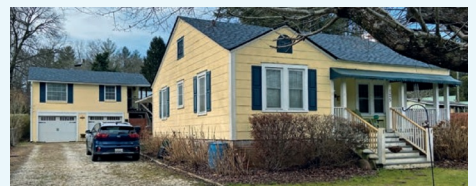
Two coach house ADUs, a type of ADU located above a rear garage, with design features that complement the single-family home.
